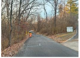
remediating the more pronounced slip would be about 188 feet and to ensure stabilization of the entire active slip area would be about 250 feet. The minimum northern limit is at the south end of the concrete driveway and the extended northern limit, to cover the entire active slip, is at the north end of the concrete driveway. Our senior engineer marked the 188-foot northern limit of the slip remediation with white paint on the roadway (see picture with painted line and paint can). The
