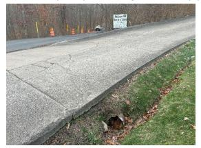
site on the north end with no evidence of recent flow of water. We could not find any inlets in the ditch on the west side of the roadway within the project area. A cross pipe was observed going underneath the concrete driveway; however, we could not find an outlet on the west side of Blackburn Road. Due to the condition of visible storm drains and some inlets/outlets not being visible, we recommend a private utility locater be engaged to map the storm drains in the area and use camera video
